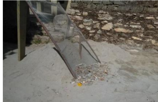
Sieving process of sand
