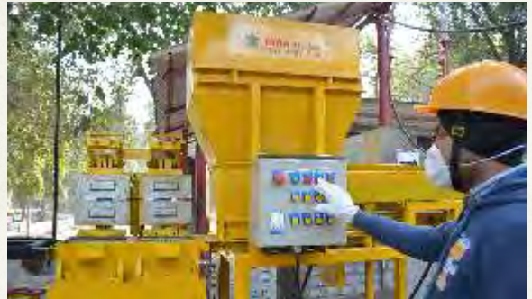
Fly ash bricks machine being operated to produce energy-efficient bricks substituting clay bricks
