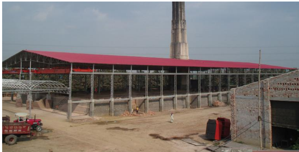
Figure 38: Natural draught Zigzag Kiln
