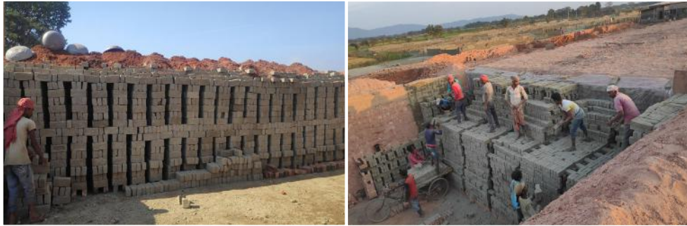
Figure 25: Brick stacking patterns during firing – FCBTK (left) and zigzag kiln (right).
