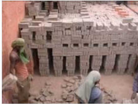
Figure 36: Stacking of unfired bricks before firing
