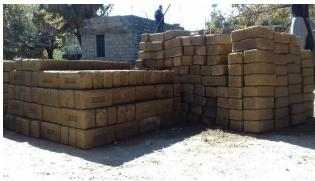
SCEB is a replacement for burnt clay bricks which are transported from more than 200 km away to rural areas. The main raw materials for SCEB – soil and coarse sand are locally available – hence SCEB are a good option for local production of masonry material. SCEB are made by compressing earth/ soil mix by simple mechanical means. The basic concept underlying compressed earth blocks is densification of the soil mix using external energy- this
