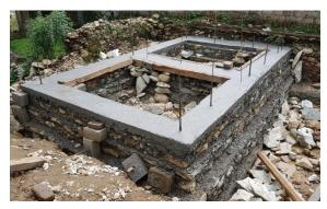
Strip footing in mortar ratio not leaner than, 1:6 is to be provided under all load bearing walls of the structure and all eccentric foundations are to be avoided. The depth of the footing is still a strata with sufficient bearing capacity. It is observed that rocky strata is found at shallow depths of 2-3 feet in most parts of Uttarkashi. A 150mm deep RCC plinth beam is to be provided across the thickness of the walls, for all load bearing walls.
