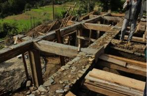
RCC columns and beams combined with traditional stone masonry in Kamad village
