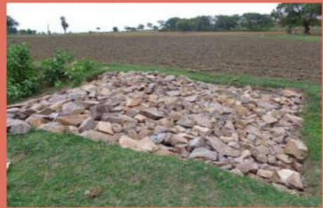
Loose boulder structure for minimizing water and soil run off
