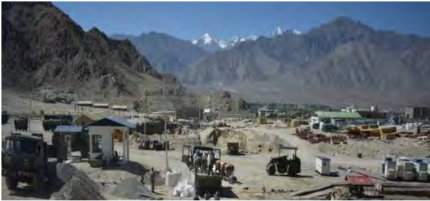
Experimental construction of heavy duty concrete pavement using LC 3 at Leh
