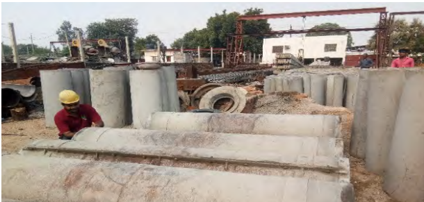
Use of LC 3 in development of hume pipes
