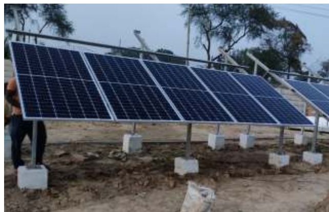
New Site at Laxmanpur Bazaar, Uttar Pradesh - Under construction
