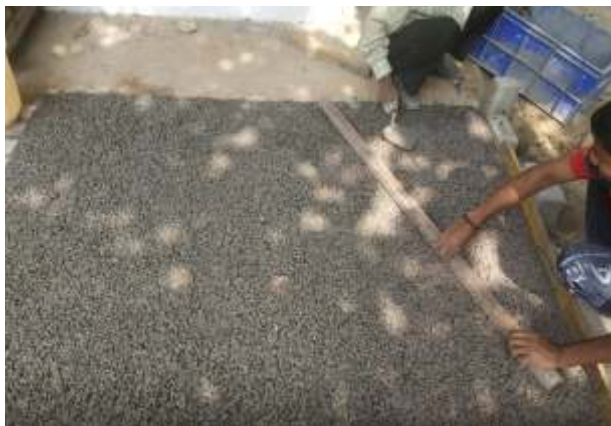
Permeable Concrete made with LC 3 Cement
