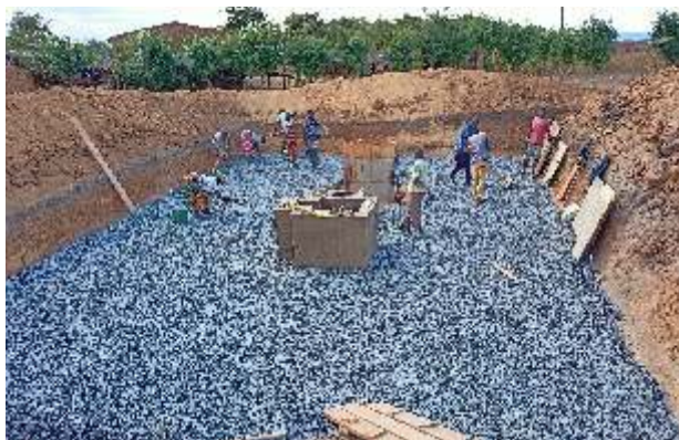
Construction of EcoKiln in Lilongwe, Malawi
